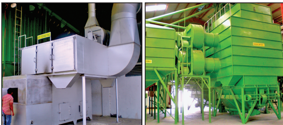
Figure 3. Scaled-up design of the multi-fuel biomass furnace (manufactured by Agri Component Corporation) retrofitted to the 30 tons capacity batch type recirculating dryers
